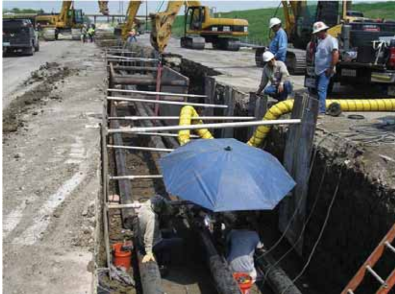
1 2 Figure 6-1. Typical HPFF Pipe Installation
