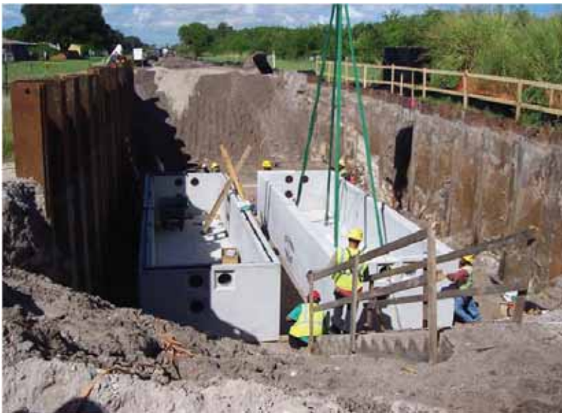
13 14 Figure 6-5. Typical XLPE Vault Installation
