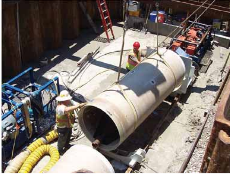
2 Figure 6-7. Typical Jack and Bore Casing Installation
